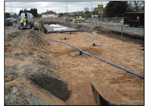
The installed top cover was just 900mm
