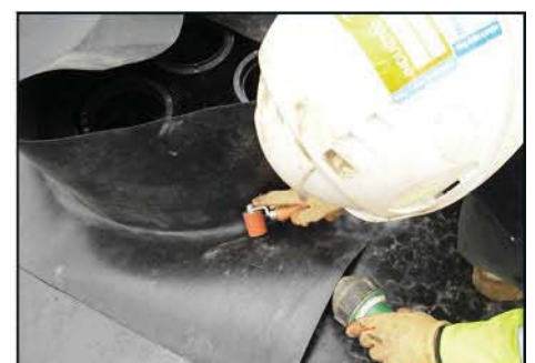
Preformed Tuflex cloaks are heat welded to inspection chamber openings.
